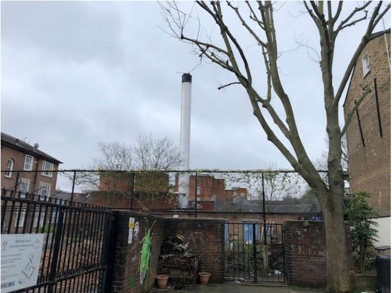
Figure 1.18: View from Crayford Road looking SW across Holloway Estate community garden to site
