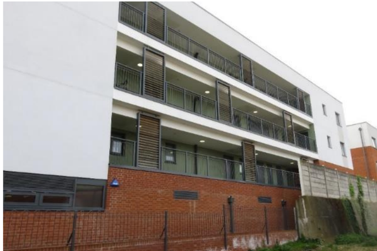
Neighbouring 275 Camden Road, showing the walkway overhangs and close proximity along the site boundary
