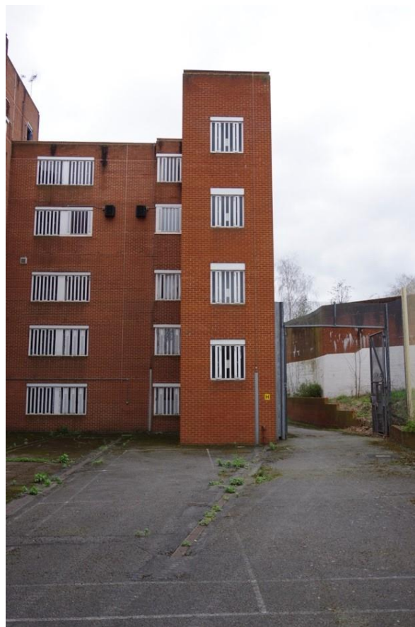
Figure 1.16: Existing buildings within the prison
