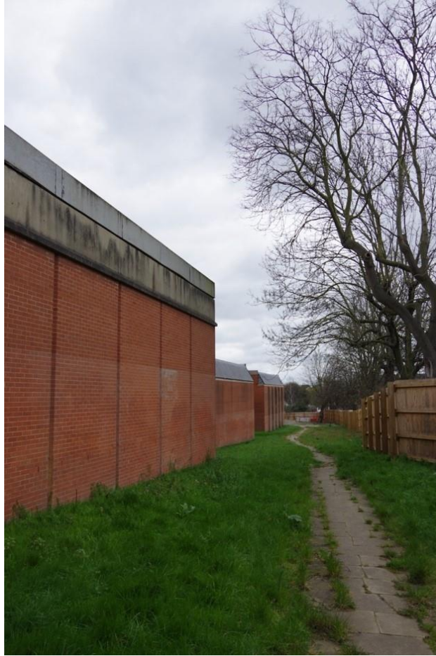
Figure 1.7: Site looking NE beyond hoarding, parallel to Camden Road
